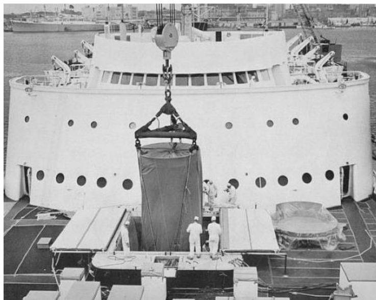
Figure 17 - NS Savannah during reactor's refuel
